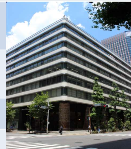
Head office: Shin-Tokyo Bldg., Marunouchi
